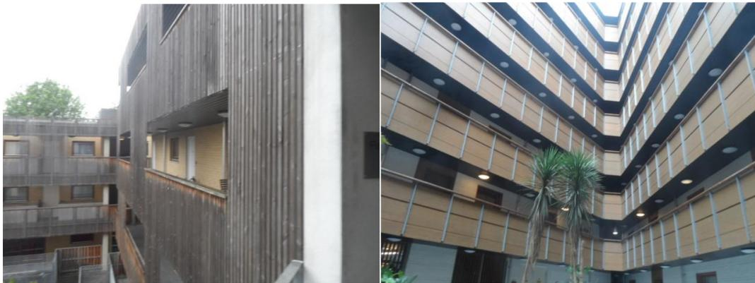
*Timber cladding in the courtyard (left) and timber balustrades in the atrium (right).*
